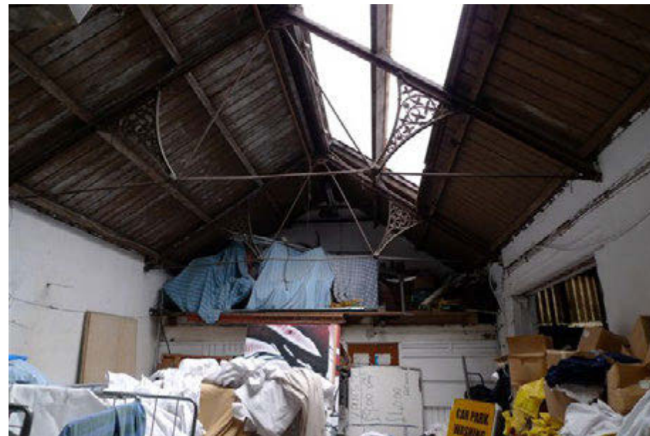
Fig 5.6.9: Mission Hall - Photograph of existing iron roof structure
